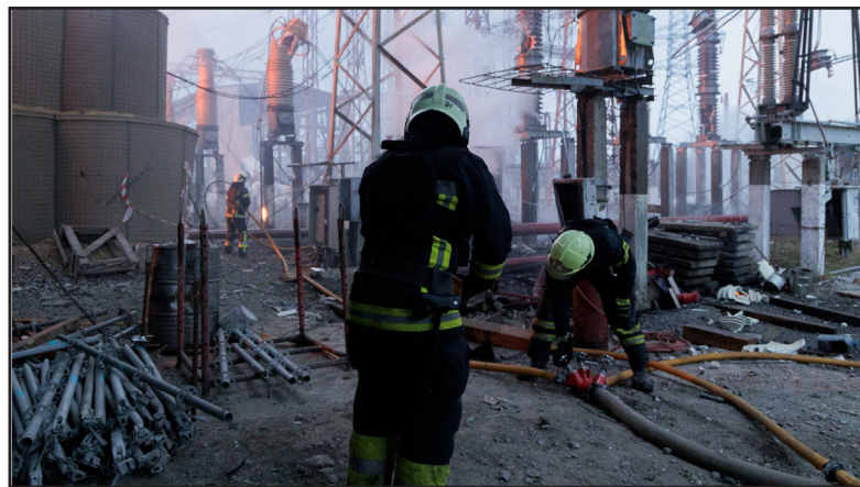
Emergency services at work in a Kyiv residential area that was struck by Russian bombs on May 8, 2024.
